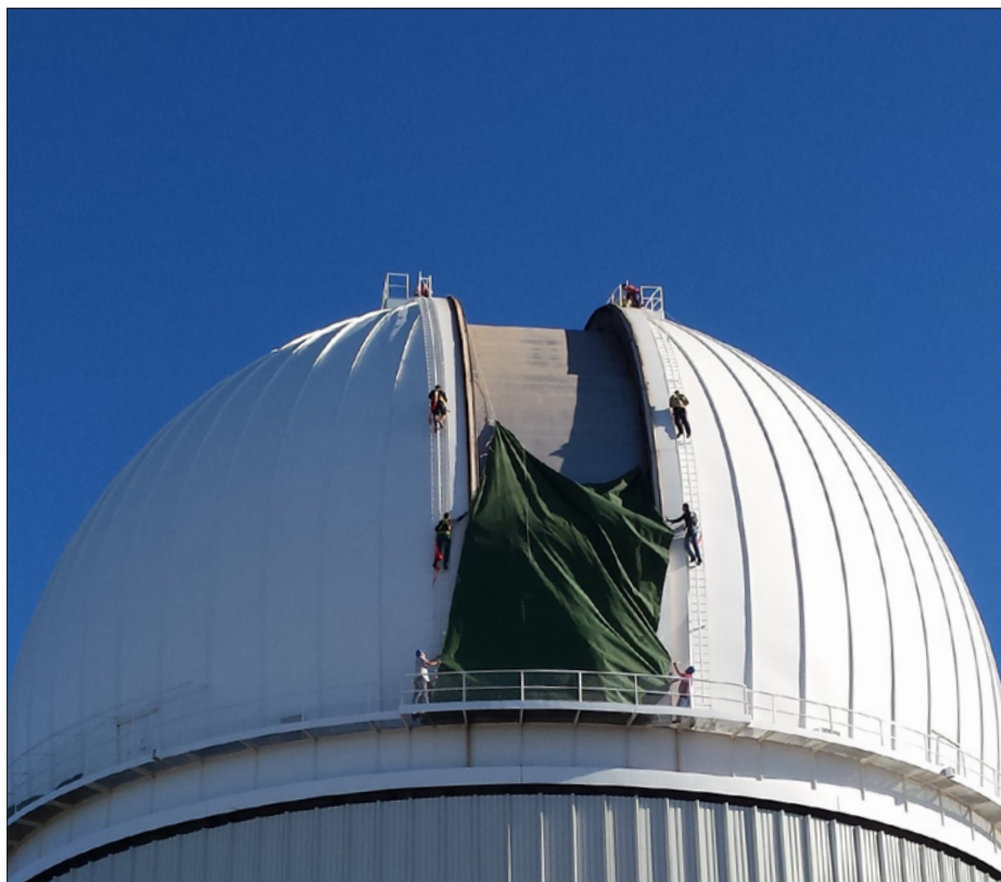
Little people on the dome: During the dome shutter repair, it was necessary to erect 2 huge tarps over the shutter to protect the interior of the dome from the elements.
